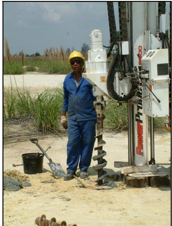
Specialist drilling on a mine slimes dam, South Africa
