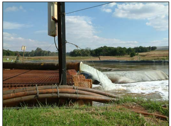
Modern-day groundwater discharge from a mine near Krugersdorp, Gauteng Province (picture: J Cobbing).
