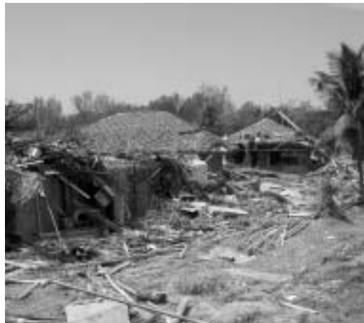
Four weeks later, these houses 250 m from the ocean at Pakwib Beach in Khaolak, Thailand, stood as the tsunami left them. The floodwater depth is clearly marked by the highest location of debris on the rooftops
