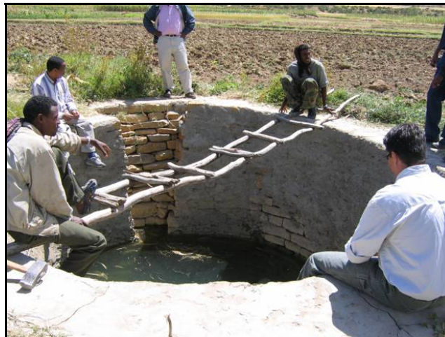
Hand dug irrigation well on the floodplain of the Berki River, Ethiopia.
