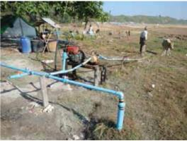
Borehole and suction pump. Water is directed through a plastic pipe to tap stands in the camp, shown in the background.
