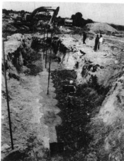
Figure 8: Completion of the continuous subsurface cutoff wall.
