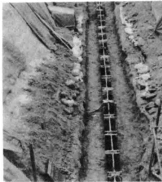
Figure 19: Completion of the subsurface cutoff wall.
