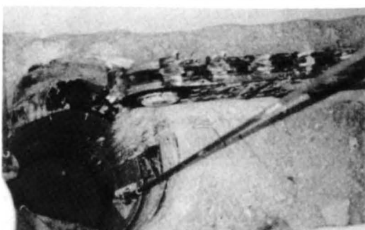
Figure 11: The chain-saw type narrow-trench excavator.
