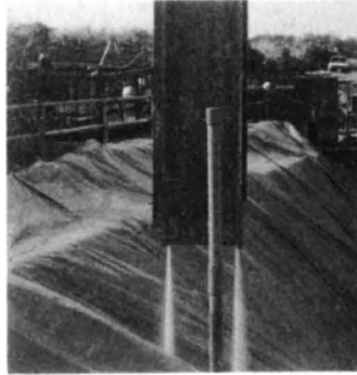
Figure 17: Testing the water jets. The water is under about 40 \text{ kg/cm}^2 pressure. Jets are located at five places on the pile.
