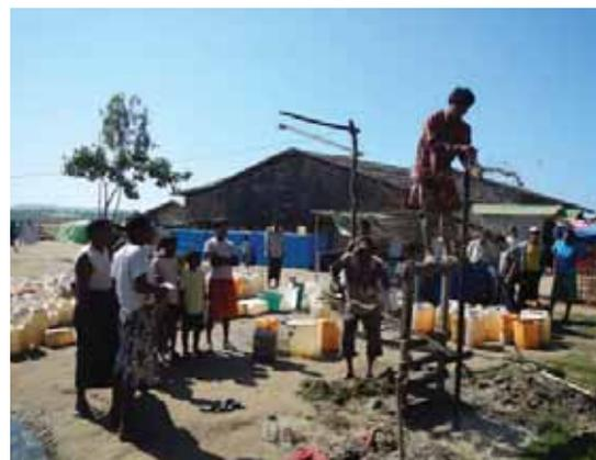
Drilling a new borehole by the sludging method in the main camp near a tapstand with water container queue.
