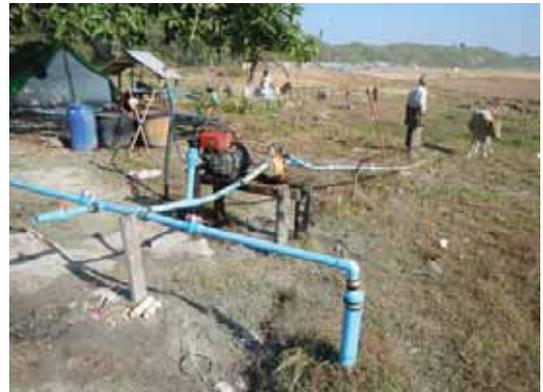
Borehole and suction pump. Water is directed through a plastic pipe to tap stands in the camp, shown in the background.
