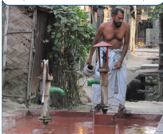
HAND-PUMP WATERWELLS IN BANGLADESH WITH GREEN SPOUT INDICATING ARSENIC-FREE GROUNDWATER (RED SPOUTS USED FOR NON-POTABLE WELLS)
