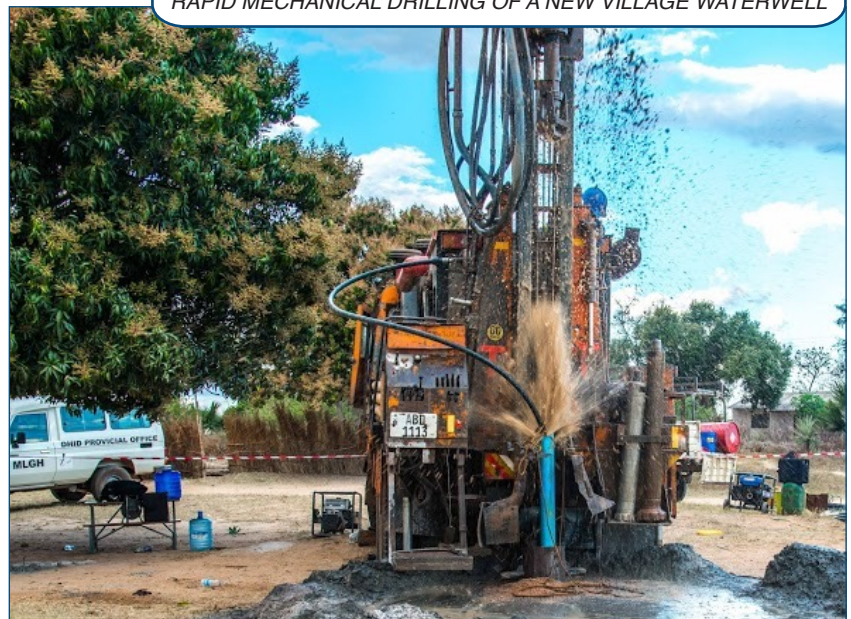
RAPID MECHANICAL DRILLING OF A NEW VILLAGE WATERWELL
