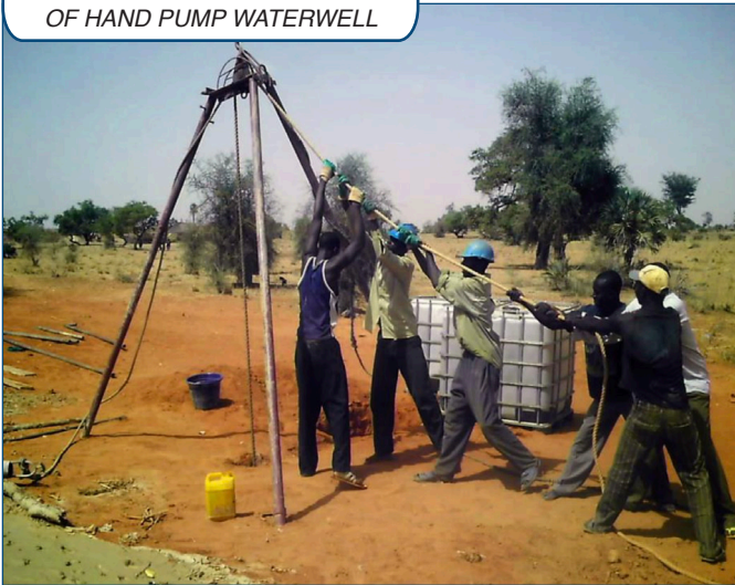
MANUAL LOW-COST DRILLING OF HAND PUMP WATERWELL
