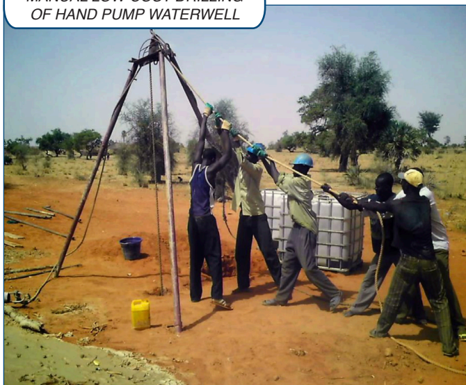
MANUAL LOW-COST DRILLING OF HAND PUMP WATERWELL
