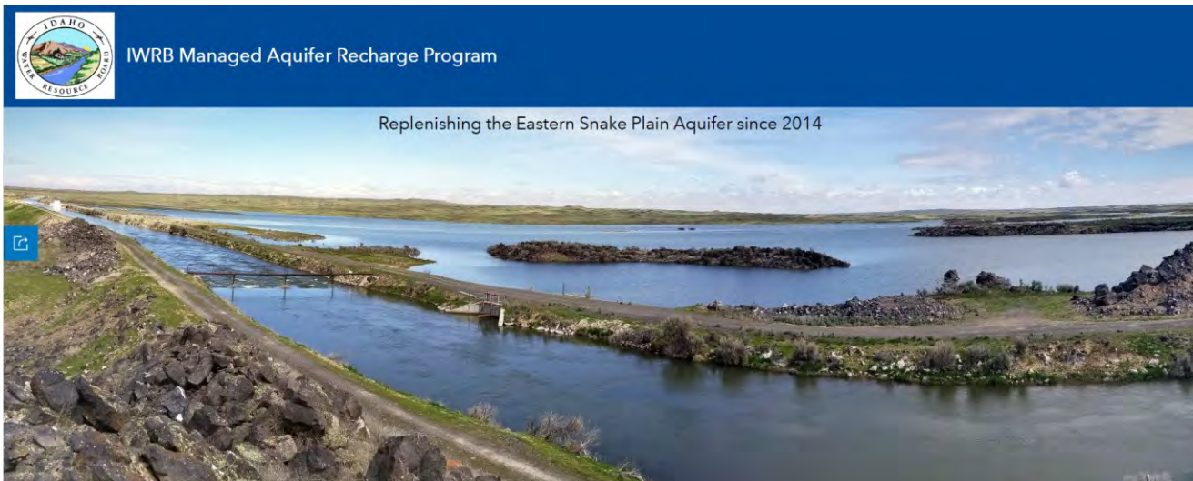
Figure 4.56 Photo of a Managed Aquifer Recharge (MAR) basin on the ESPA, Mile Post 31 behind the Milner-Gooding Canal from April 2019. Mile Post 31 (MP31) is one of the major first milestones of the IWRB's MAR program. The IWRB partnered with AFRD#2 to construct the MP31 site completed in 2013. The original turnout structure was designed for 200 to 250 cfs. Using this structure only inundated approximately half of the available basin. In 2016 a second turnout structure was constructed consisting of an obermeyer weir and headgate structure. This allows for water to be raised in canal and diverted into the basin. The site can infiltrate upwards of 650 cfs of water. Due to canal improvements at the MP28
