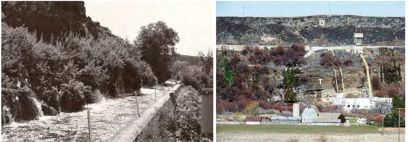
Figure 4.31 Left: Thousand Springs flume. Springs emerge from pillow lavas of Thousand Springs Basalt at left. Flume is constructed on the Banbury Basalt. Spring water is transported by the flume to an electrical generating plant that has been in operation at this site since 1911. The photograph shows part of spring location number 1 in Figure 4.32. From Covington and Weaver, 1991. Right: Thousand Springs Power Plant. Q: Quaternary Thousand Springs Basalt (pillow lavas); T: Tertiary Banbury Basalt (low permeable). From Farmer, 2021.
