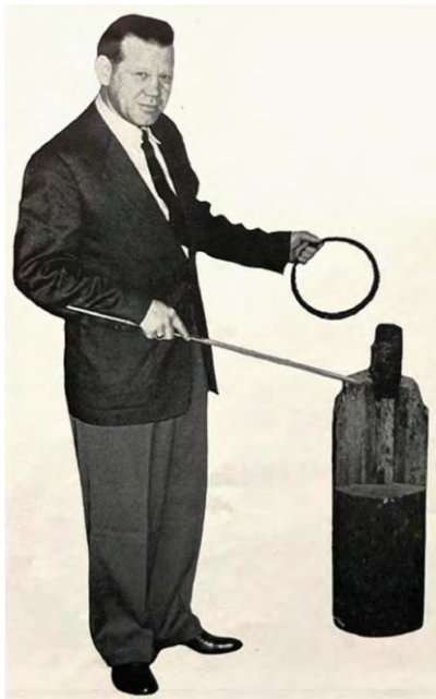
Figure 8.37 A section of the original wooden pipe laid in Winchester in 1808. Mr. S. L. Grant, Winchester City Manager, shows how the log pipe was fastened together. The iron sleeve (to which he is pointing) was on the inside while the iron ring (which he holds in his left hand) was on the outside. From Lemon, 1955.
