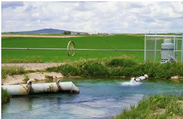
Figure 4.50 The Snake River Plain basalt-rock aquifer supplies large volumes of groundwater from great depths for irrigation. Here, a single well produces over 1,000 gallons of groundwater each minute to irrigate the surrounding fields. There are over 100 of these irrigation wells in the A&B area of the Snake River Plain where groundwater is pumped and applied to crops, and then excess irrigation water is recharged back to the groundwater. This cycle causes dissolved constituents, such as salts and nitrate, to become more concentrated. Photograph by Charles D. Hunt, USGS. From Rupert et al., 2014.
