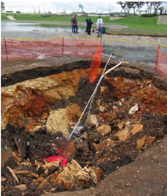
Figure 5.14 On January 24, 2012, a 4.5-inch rainfall filled a Storm Water Retention Pond (SWRP) located in the recharge zone of the Barton Springs segment of the Edwards Aquifer with about 10 feet of stormwater. Subsequently, a cover-collapse sinkhole developed within the floor of the SWRP, measuring about 30 ft in diameter and 12 ft deep. About 7 million gallons of stormwater drained into the aquifer through this opening. To determine the path, velocity, and destination of stormwater entering the sinkhole, a dye trace was conducted. Phloxine B was injected into the sinkhole on February 3, 2012. A mass of 16.27 lbs (7,382g) was mixed with water and then gravity injected via a hose using storm water from an adjacent pond.
