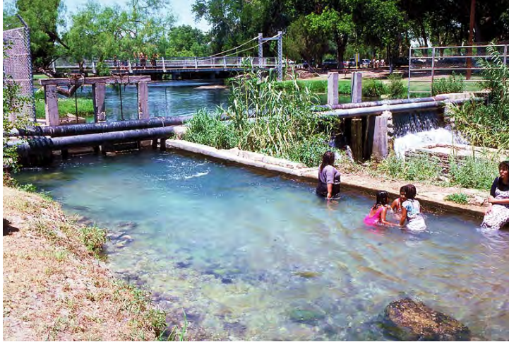
Figure 5.49 Blue Lake, early 1990s. Water leaving Blue Lake, which is fed by Springs 1, 2, and 4. Discharge from the Lake is split: water flowing to San Felipe Creek is running over the spillway on the right, and the Acequia Madre Canal is on the left. Photo courtesy of Gregg Eckhardt.
