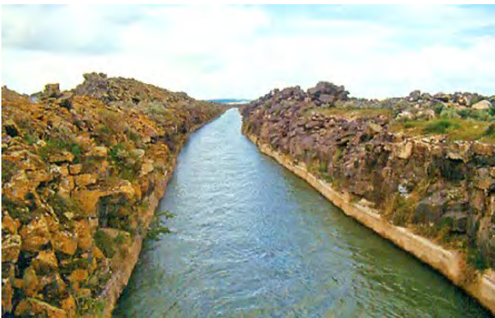
Figure 4.52 Extensive irrigation canal systems divert water from the Snake River and distribute it across the Snake River Plain to irrigate fields. The Northside Canal, shown here, is located near Milner Dam where, depending on season, the entire flow from the Snake River may be diverted for irrigation. Photograph by Michael G. Rupert, USGS. From Rupert et al., 2014.
