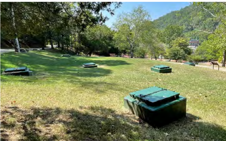
Figure 9.52 The bulk of the thermal water flowing each day from Hot Springs Mountain is collected from 27 of the 47 presently active springs. Each spring in the collection system has been sealed and covered with a green box about four feet square with a metal cover, chain, and padlock. The green boxes on the lower west slope of Hot Springs Mountain and the heat exchange units at the north end of Bathhouse Row are the most visible components of the thermal water collection and distribution systems and represent its source portion. Not all the boxes indicate a spring; some hold only valves and collection plumbing.
