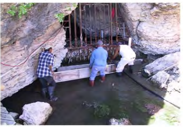
Fig. 5a – installing concrete forms
