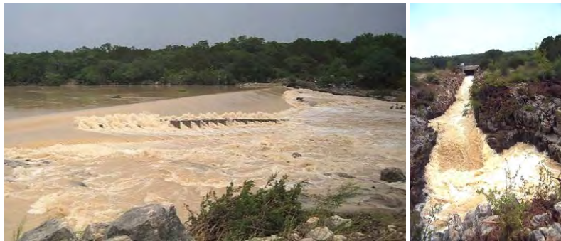
Figure 5.5 Edwards Aquifer recharge dam on Seco Creek. Part of the flood water is diverted towards the Valdina Sinkhole, shown on the right photo, via artificial channel incised into Edwards Limestone. Courtesy of Edwards Aquifer Authority.
