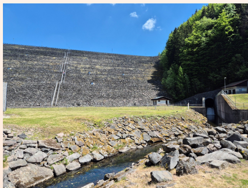
Turcek drinking water reservoir (photo Katarina Benkova)
